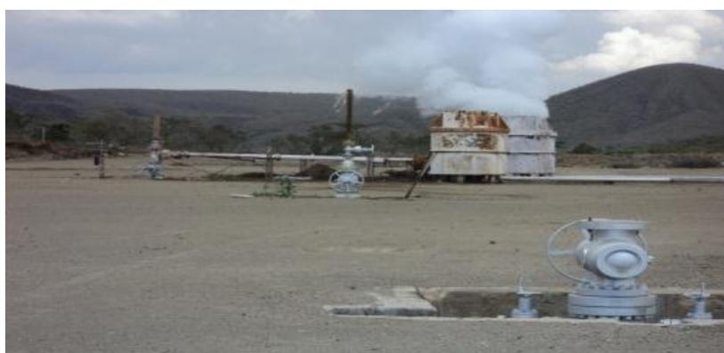
Figure 5. Pad #915 hoisting three wells
