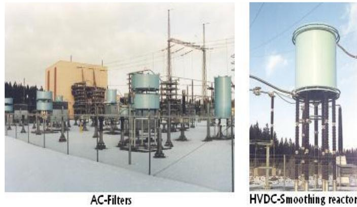
fig. HVDC Smoothing Reactor
