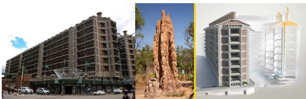
Cool air enters through the lower parts of the building and is circulated by fans, the air becomes warmer and lighter as it rises through the various floor of the building, and finally escapes through chimneys at the top of the building. The natural system helps reduce energy consumption by 10% when compared to a standard
