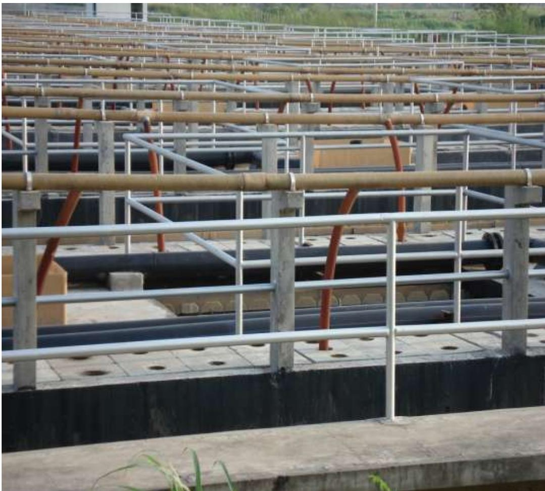
**Fig 1.2:UASB Reactors**
