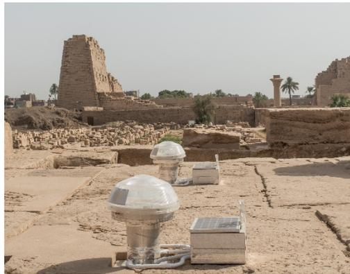
**Photo 21:** Solatube ® domes with solar powered ventilation
