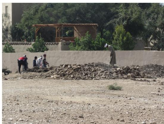
**Photo 8:** Mud brick debris after sorting. Designated for recycling
