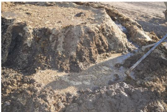
**Photo 10:** Mixing the mud brick debris with water and straw as needed
