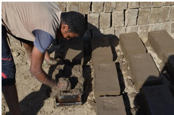
**Photo 11:** Placing the recycled mud brick debris in the mold. Forming and stamping with mission's logo
