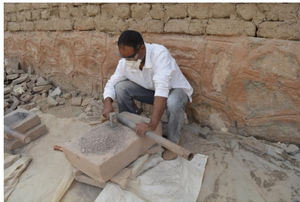
**Photo 17:** Crushing scrap stone to power to be used as an ingredient in lime mortar
