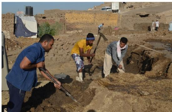
**Photo 9:** Mud brick debris broken down to start the mixing process
