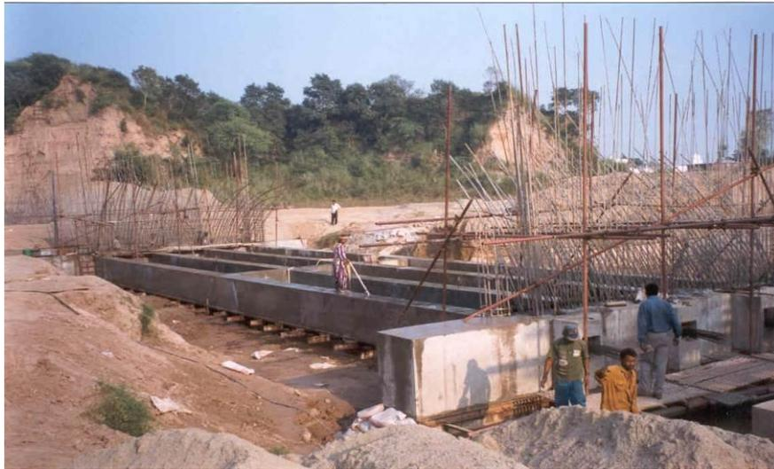
Photo.2. Construction of prestressed tie beams at springing points under progress
