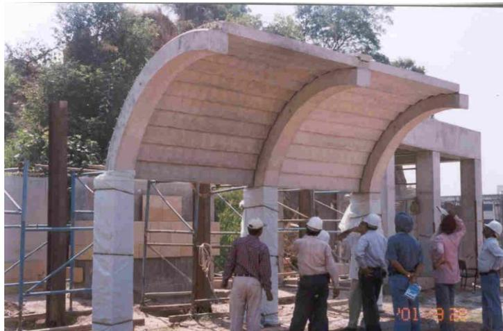
Photo.6. Mockup of three pieces of precast canopy to simplifying handling
