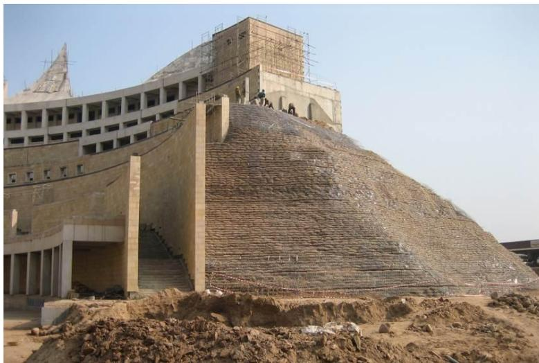
Photo.13. Remaking of hillocks using geogrids as soil reinforcement
