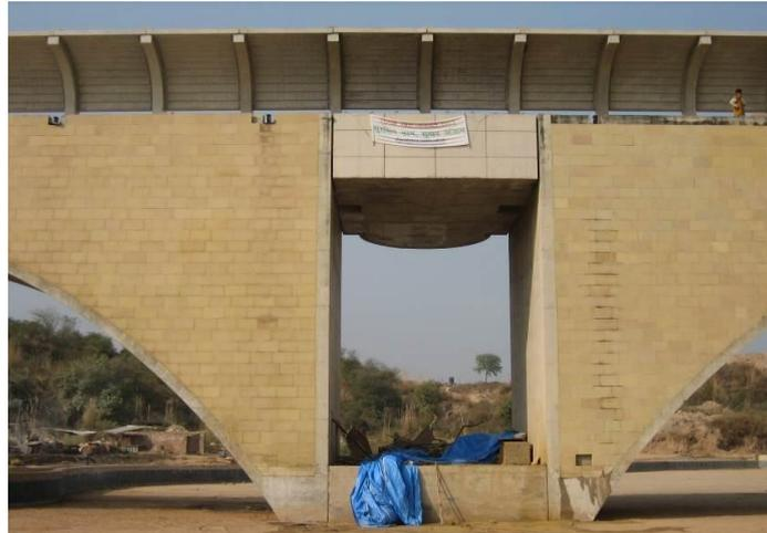
Photo.3. Independent slab separating two arch bridges
