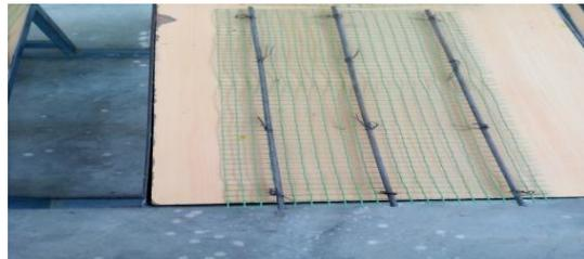
FIG.3.8: MESH WITH SKELETAL STEEL
