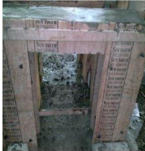
Figure 8(b) Casting of frames
