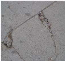
figure 7 Corner crack
