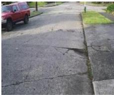
figure 3 Corner crack
