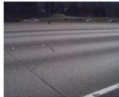
figure 4 Corner crack
