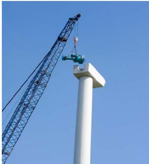
Fig 2.-Wind Turbine Gearbox Installation
