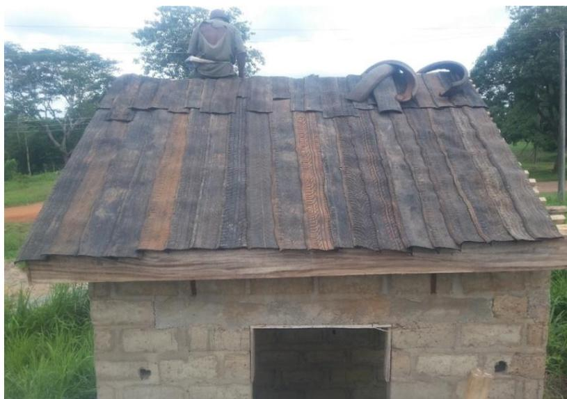
**Plate1:** The Constructed Tyre Roof
