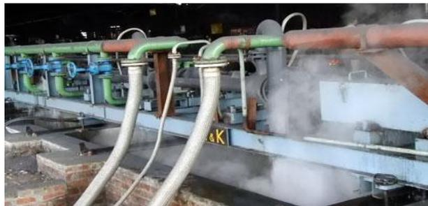
Fig.2: Shows water pressure control valve in cooling system
