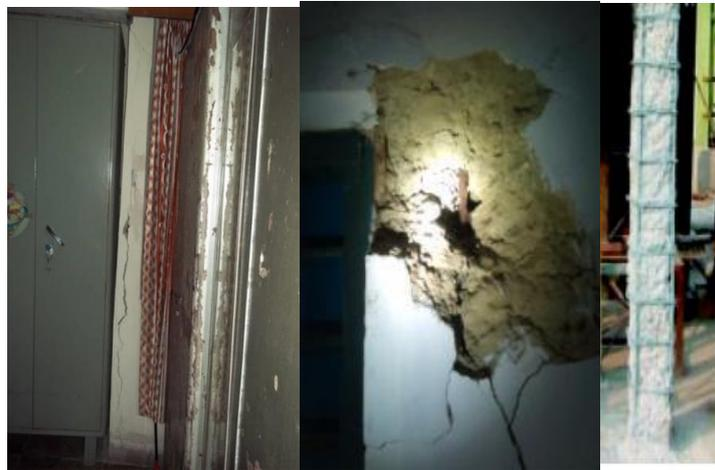
**Fig.3. Damaged column a) and b) Before removal of cover concrete and c) After removal of cover concrete**
