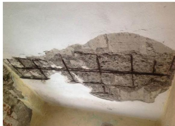
**Fig: 13 Damaged Slab**
