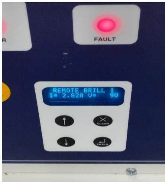
Figure 9. Test results on CCR display
